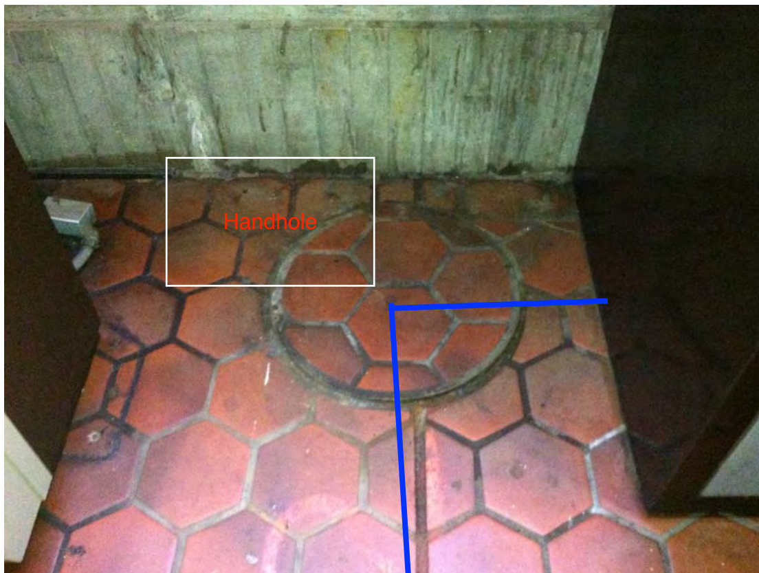
Photo #2 – Handhole adjacent to fare vending machines on mezzanine floor
